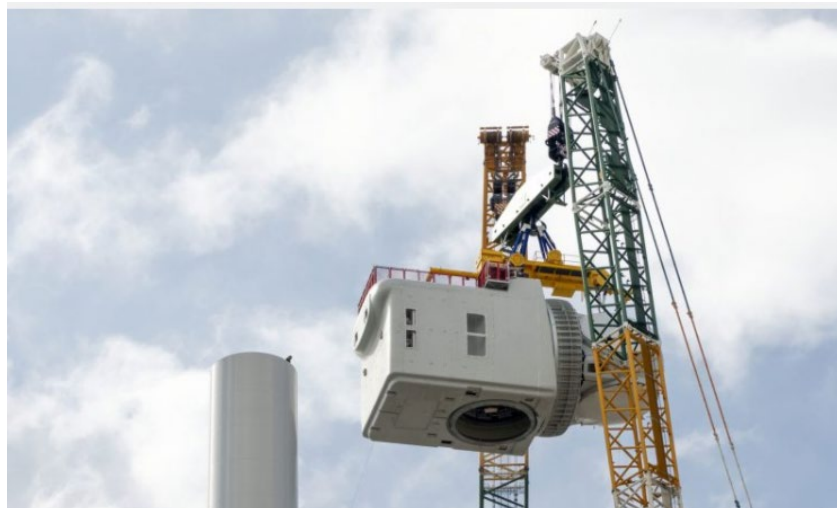
Figure 11 Installation of the 570 MT, GE 12.5MW Prototype by Dual Lift (Source: GE Renewable Energy)
