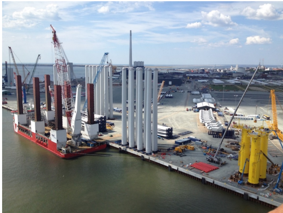
Figure 14 Wind Towers Being Loaded Out (Source: MHI Vestas)
