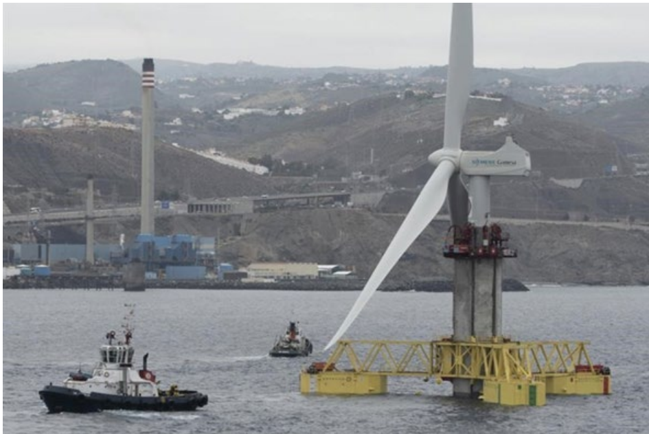
Figure 20 Estyco Elisa Being Towed to Location (Source: Elican Project)
