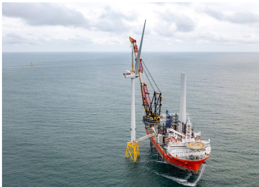
Figure 16 Offshore Blade Installation (Source: SSE Renewables)
